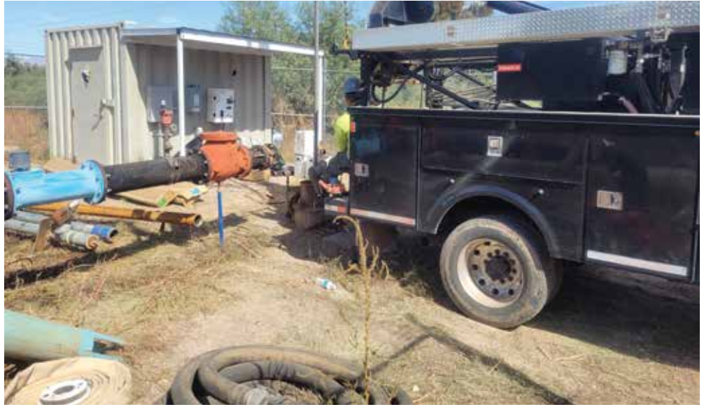
WELL WORKERS CLEANING AND DISINFECTING THE NORTH WELL TO ADDRESS WATER QUALITY CONCERNS
