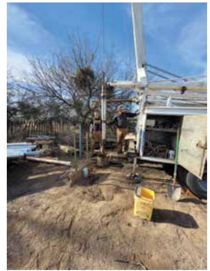
WELL WORKERS INSTALLING A TEMPORARY PUMP FOR WASH WELL DURING TESTING.
