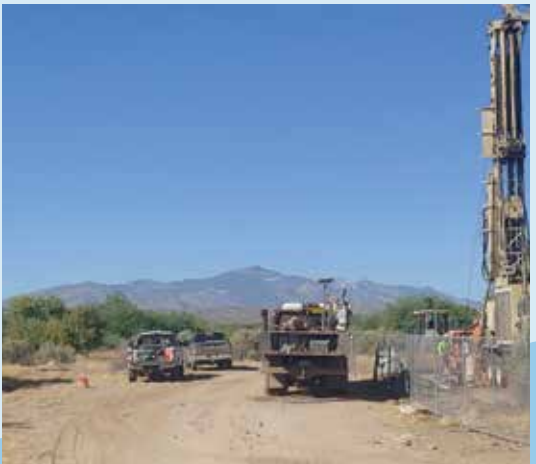
DRILL RIG CREW DRILLING A NEW IRRIGATION WELL AT GOODWIN WASH.
